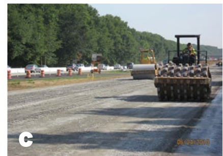
Figure 6.3 Rubblization of JRC: a) Installation of geocomposite edge drain, b) Rubblization of JRC, and c) Compaction of rubblized JRC (Courtesy of NJDOT)
