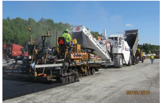
Figure 6.4 Construction of BRBC Layer over Rubblized JRC (Courtesy of NJDOT)
