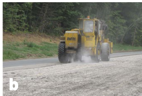
Figure 6.3 Rubblization of JRC: a) Installation of geocomposite edge drain, b) Rubblization of JRC, and c) Compaction of rubblized JRC (Courtesy of NJDOT)
