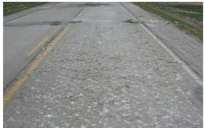
b. Modified Rubblization
