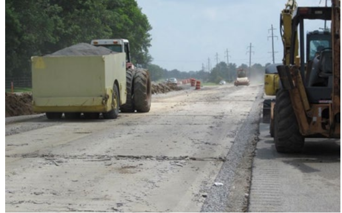
b. Seating after Breaking
