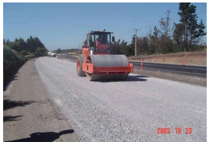
b. Compaction with a Smooth Steel Roller
