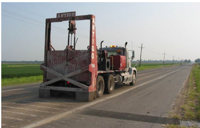
a. Cracking Operation for C&S
