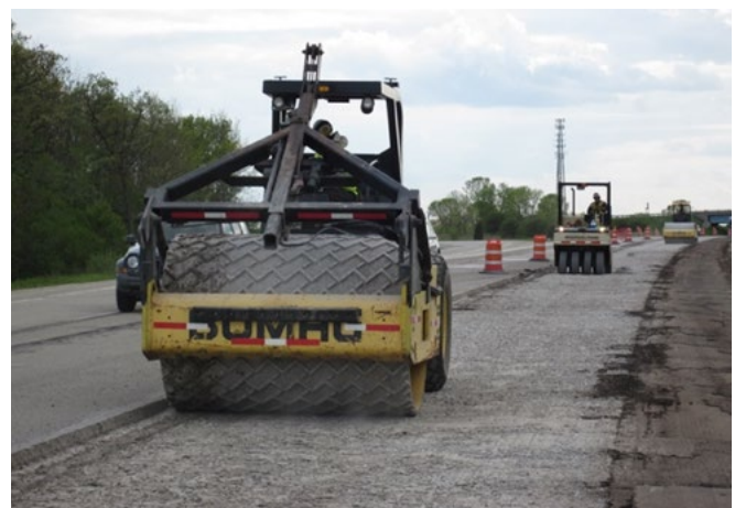
b. Three-Roller Compaction Process
