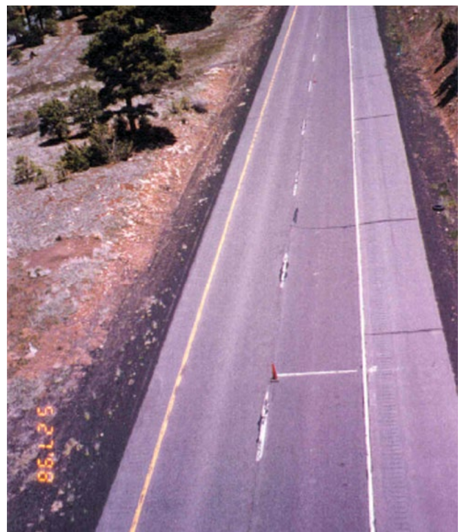
Figure 5.4 I-40 SHRP Test section nine years after construction: conventional asphalt concrete (left) and asphalt rubber concrete (right) (Way 2000b)
