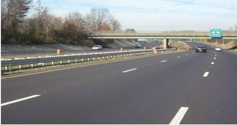
Figure 6.5 I-295 Perpetual Pavement after 10 Years of Excellent Performance (Courtesy of NJDOT)
